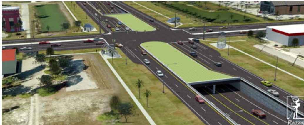
Figure 13: Arterial Underpass Queue Jump
