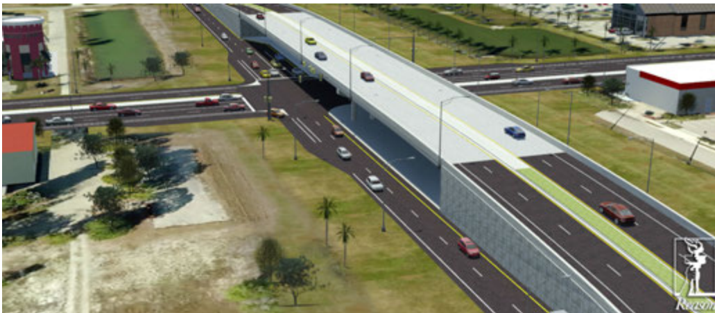
Figure 12: Arterial Overpass Queue Jump
